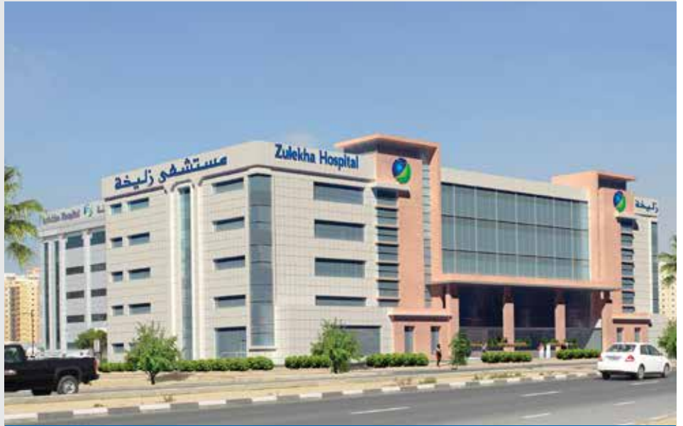
Zulekha Hospital – Cancer Care Center, Dubai
